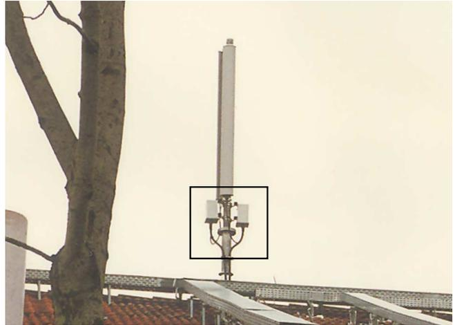
Photo 16: Subsequently installed tower mounted amplifier (TMA) between connecting cable and feeder cable
