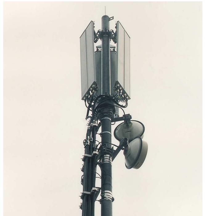
Photo 2: Two antennas per sector. Installation of 2 F-Panels per sector using 2 x F-Panel Mounting Kits.
