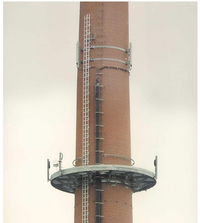
Photos 10 and 11: Installation of an antenna platform at a height of approx. 50 m with the help of two auxiliary platforms.
