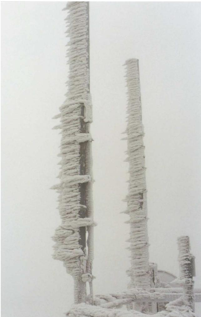
Photo 3: Iced up Kathrein omni-directional antennas – fully functional!
