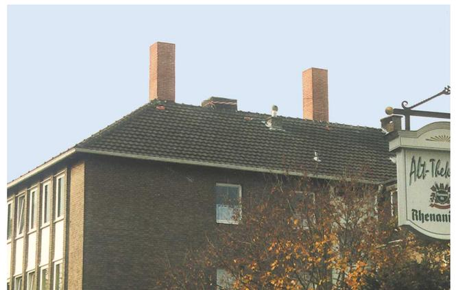
Photos 19 and 20: Antennas completely disguised (Source: NAUTICO-GFK-Produkte-GmbH, D-45869 Gelsenkirchen)
