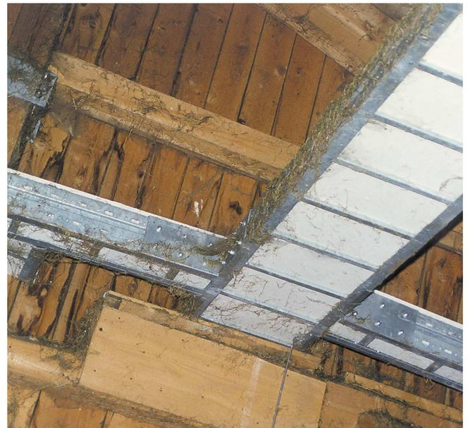
Photo 24: Fire protection of a cable path rinne in a shed barn, in accordance with fire protection class F90.
