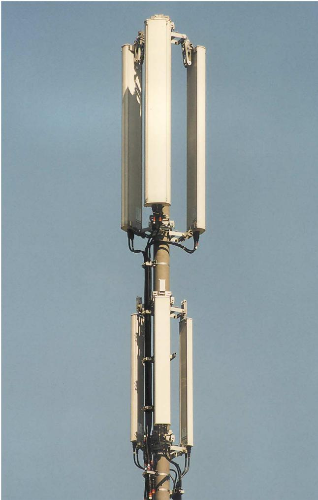
Photo 12: Cable led upwards behind antennas mounted at a distance.
