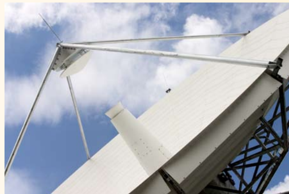
Fig. 1: 9.5 m C-band antenna installed at Munich site
