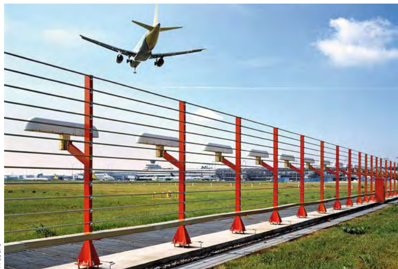
FIG 3 ILS systems of the III b category require high-precision measurement instruments for checking the DDM values.
