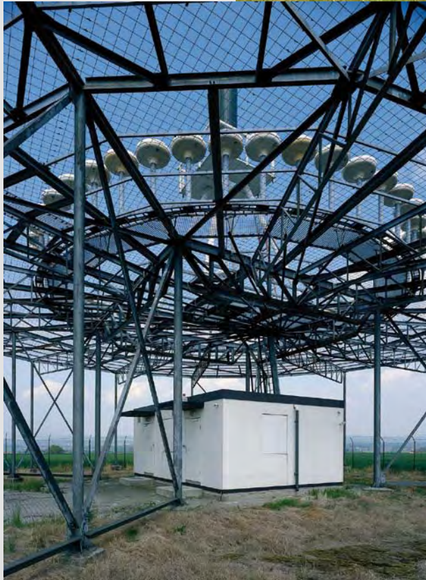
FIG 5 When checking CVOR/DVOR antenna systems in accordance with ICAO Doc. 8071, the R&S®EVS 300 analyzes both useful and spurious modulation.
